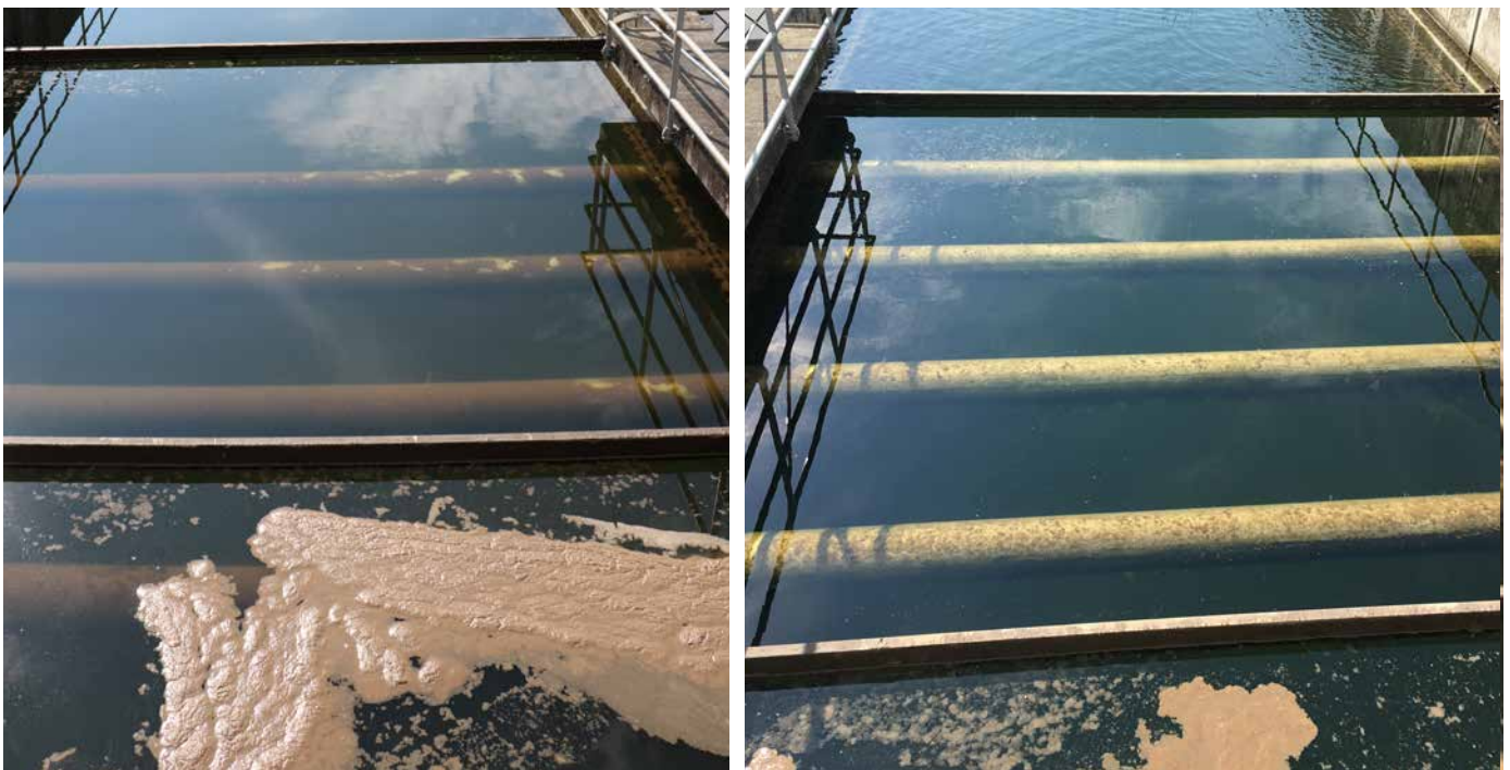
Depth of visibility and turbidity respectively in the secondary clarifier Left: untreated; right: treated with VTA Hydroprompt® FORTE after 24 hours.
