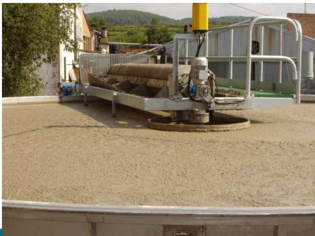
**FLOTADOR DAF POR AIRE DISUELTO
