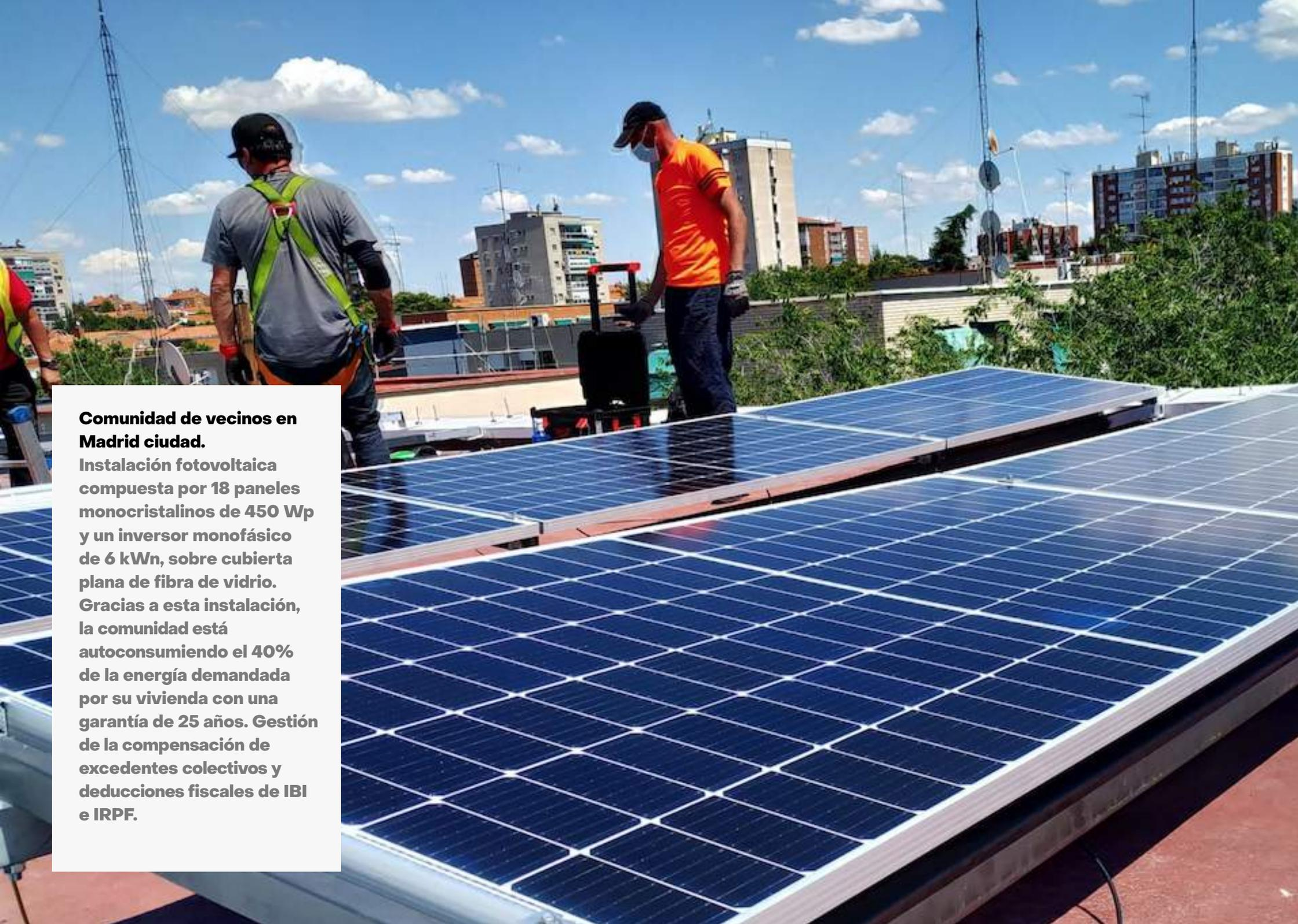
A photograph showing two workers on a rooftop installing solar panels. One worker in a grey shirt and safety harness is in the foreground, and another in an orange shirt is further back. The roof is covered with rows of blue monocrystalline solar panels. In the background, there are city buildings and utility poles under a blue sky with scattered clouds.
